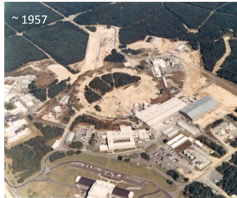
AGS construction, Brookhaven, New York
