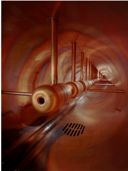
DTL tank - Fermilab
